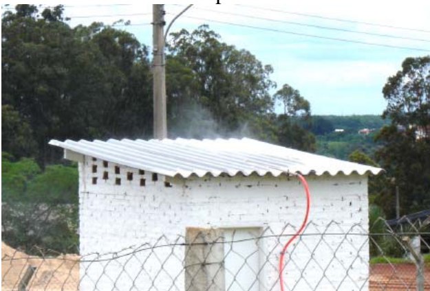
Figure 4 – Passive cooling – water spraying on roofing.
